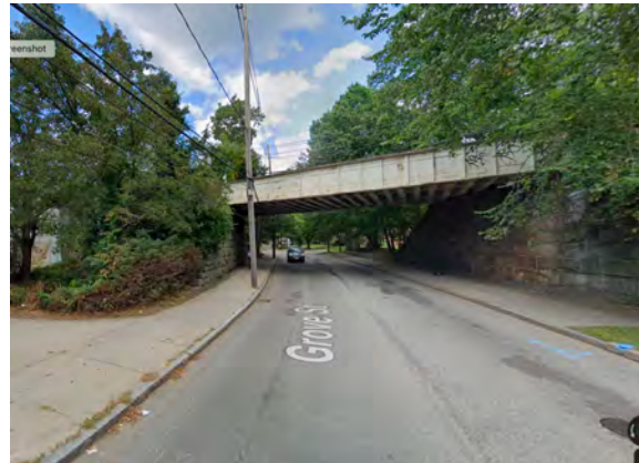
Figure 6. Grove St south of railroad overpass.
